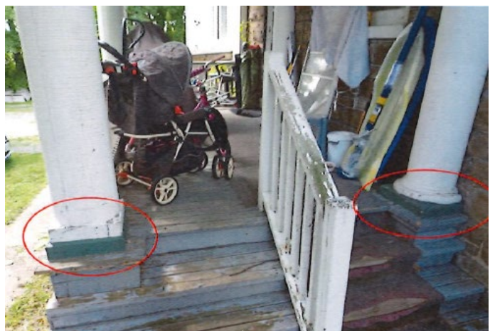
Figure 9 East side porch columns failing
