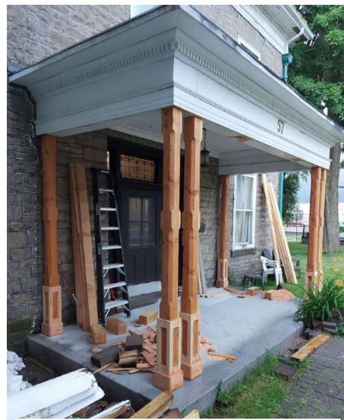
Figure 7 - columns the owner has installed using Douglas Fir lumber from Peterborough.
