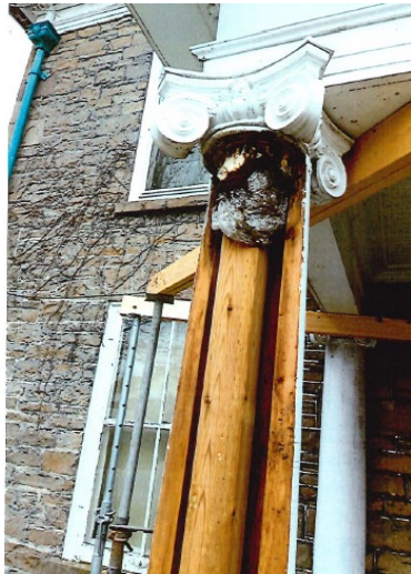
Figure 3 - rotted column at top
