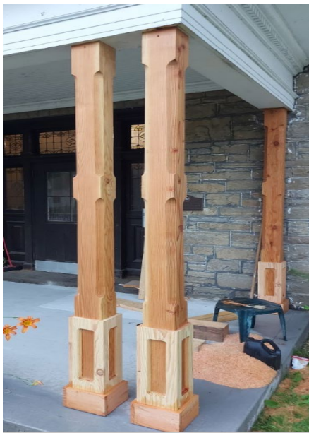
Figure 6 - columns the owner has installed using Douglas Fir lumber from Peterborough.
