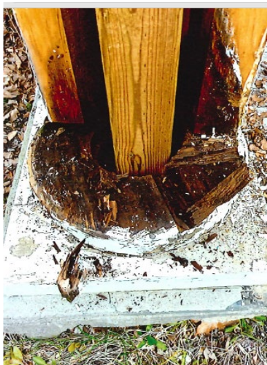
Figure 2 - rotted column base
