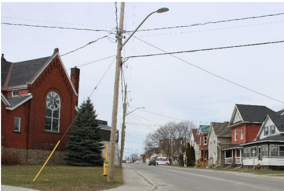
Photo 6.12 Streetlights on wooden utility poles, looking north on Elmsley Street North
