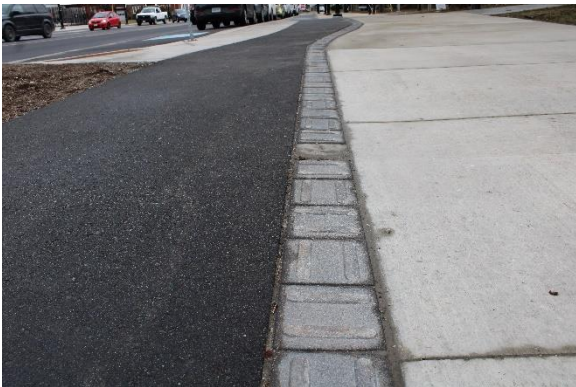
Photo 6.6 Strip of decorative interlock paving beside bike lane along Beckwith Street, looking north
