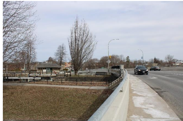
Photo 6.4 Bridge along Beckwith Street, looking northeast (away from the Study Area)
