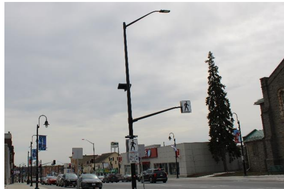
Photo 6.11 Utilitarian streetlights along Beckwith Street, looking south
