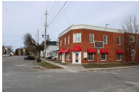
Photo 6.7 Grassed boulevard along Main Street West, looking west
