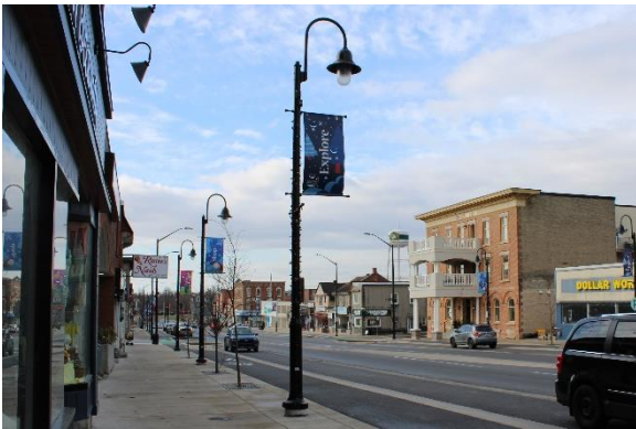
Photo 6.10 Decorative Streetlight along Beckwith Street, looking south
