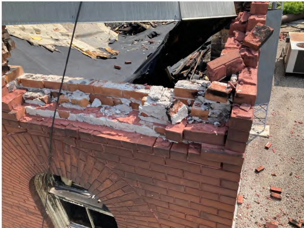
RE8 Brick Parapet
