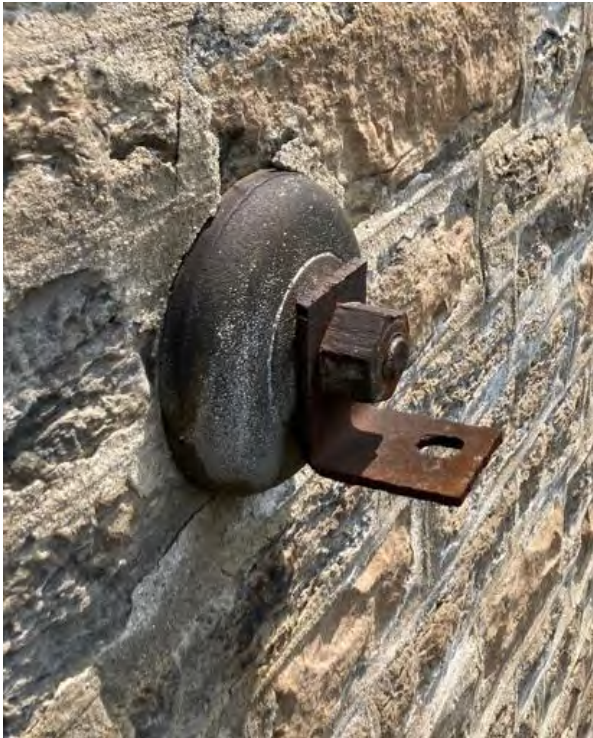
Fig 15. Through-bolt wall anchor at 3E2.
