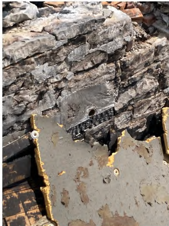
RC5 1868 exterior 1896 interior
