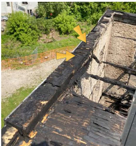
Fig. 10 Concave parapet at RE3.
