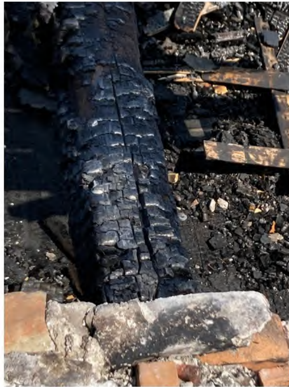
RC5 Timber roof beam
