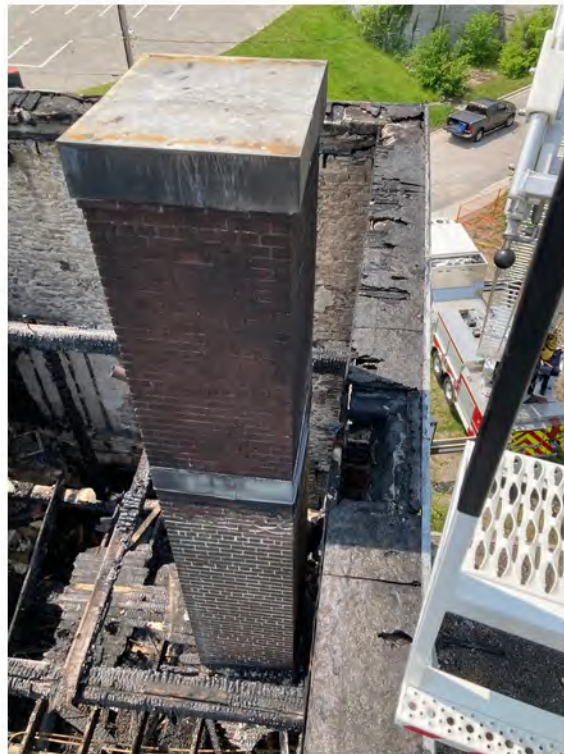
RC1 East face of chimney
