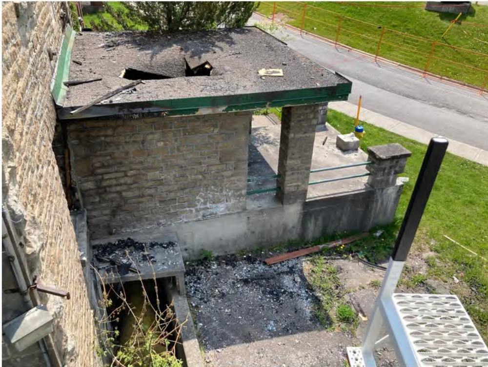
Entrance Addition north elevation and roof
