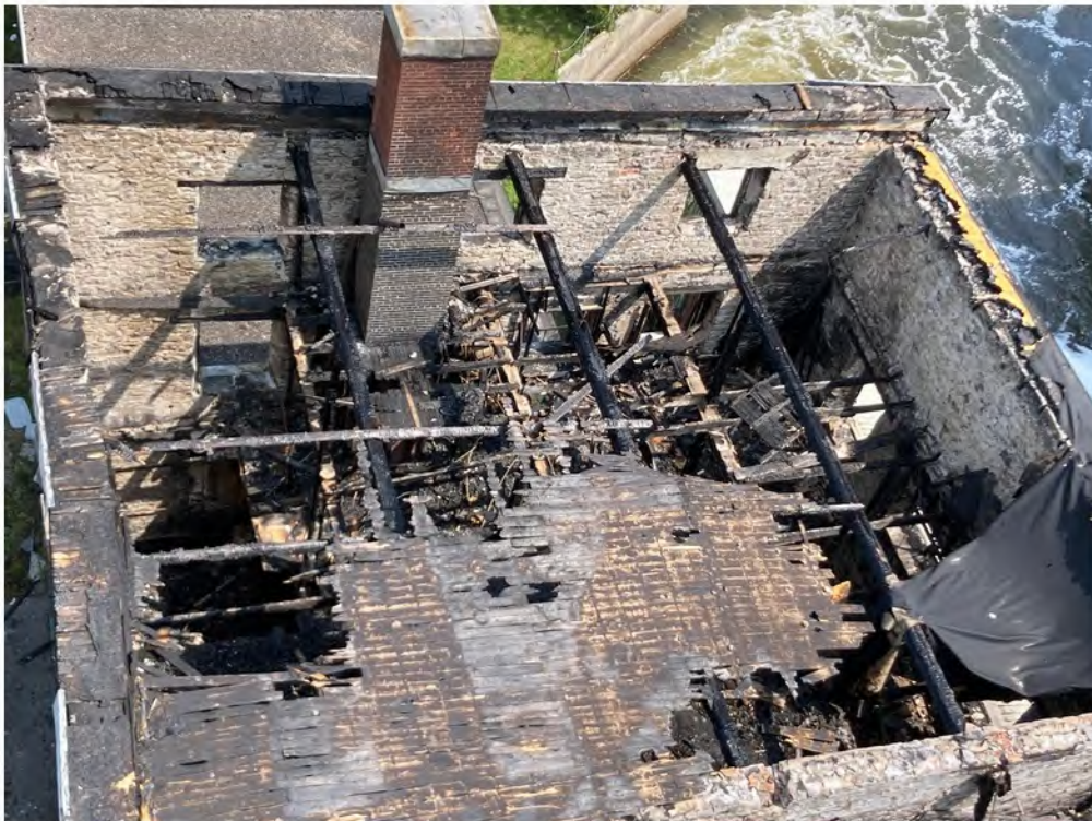
RE1-RA1 to 2E1-2A1 interior
