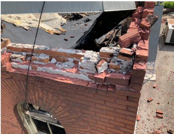
Fig 19. Building 3 is triple wythe brick masonry.
