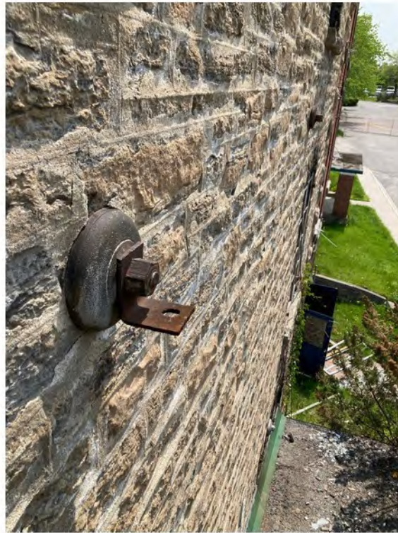
E3 bell tie-back at 3rd floor elevation
