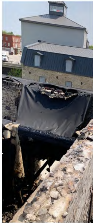
RA4-RA5 roof membrane
