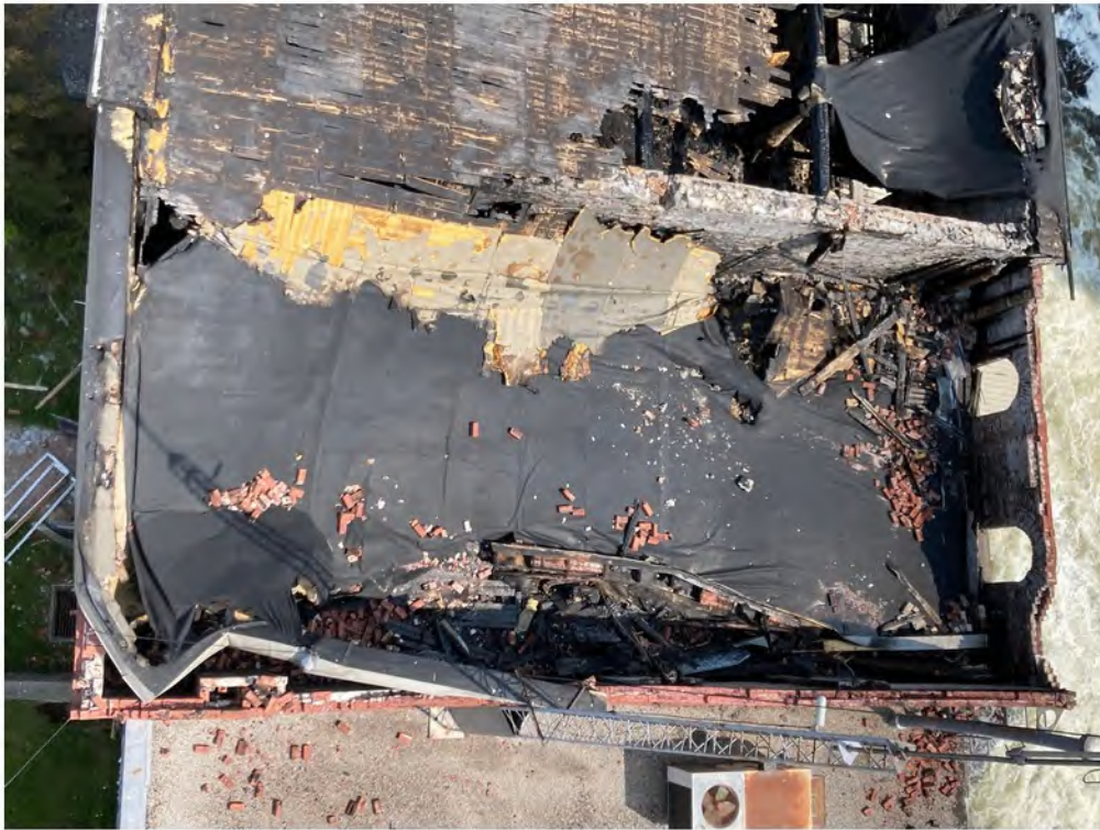
Aerial View 1896 Brick Bdg Roof
