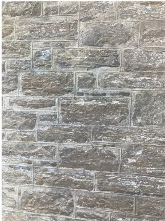
2D1 exterior good condition
