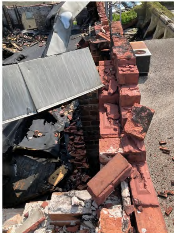
E8-D8 Brick Parapet
