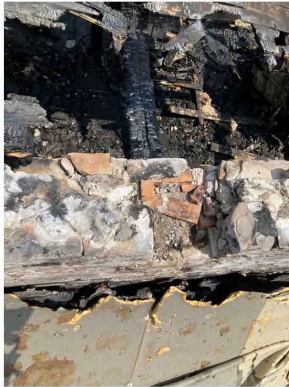
RC5 Parapet sample location
