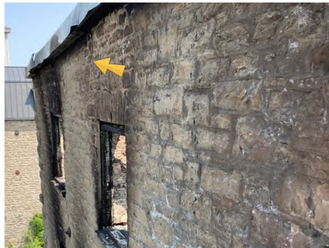
Fig.11 Convex parapet at RB1.
