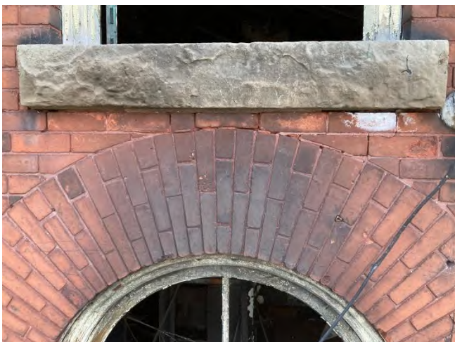
Fig 17. Brick voussoir and sill at 3E6.5.
