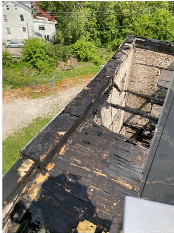
RE5-RE1 aerial interior
