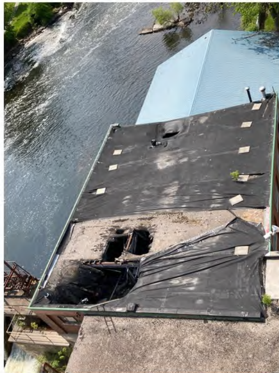
Aerial View 1924 Bdg Roof
