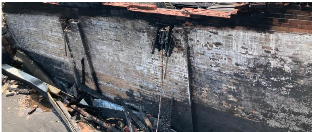
Fig 14. Plaster parging evident on the interior face of 3A8-3E8.
