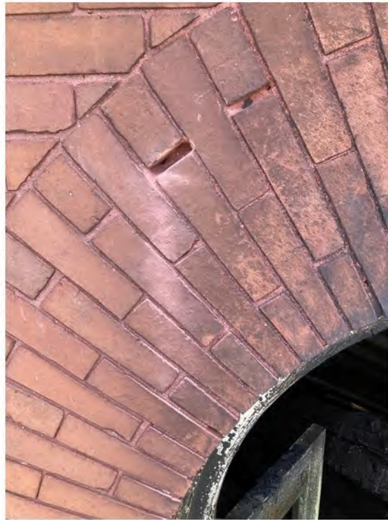
3E6.5 red brick mortar sample locn
