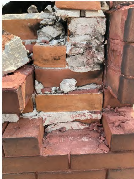
RE8 Brick Parapet sample locn
