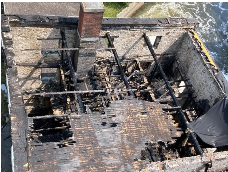
Fig 21. Aerial view of Building 2 interior.
