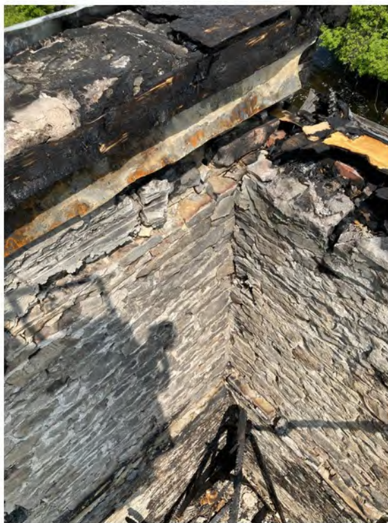
3A1 interior corner
